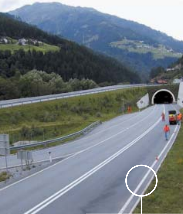
Low-cost road markings with increased retroreflection and profiled actions reduce the number of accidents, in particular involving collision with tunnel portals. Photo: Swarco
