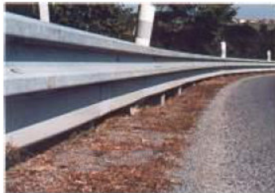
Figure 2. The Plastrail by Solidor. This plastic covering provides protection to motorcyclists by covering the posts of the guardrail (Limi et al., 2008).
