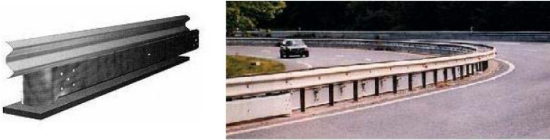
Figure 1. Metal shield developed by SEC-Envel. The flexible metal covers the hazardous posts and prevents motorcyclists from colliding with them (FEMA, 2000 [left] and Limi et al., 2008 [right]).
